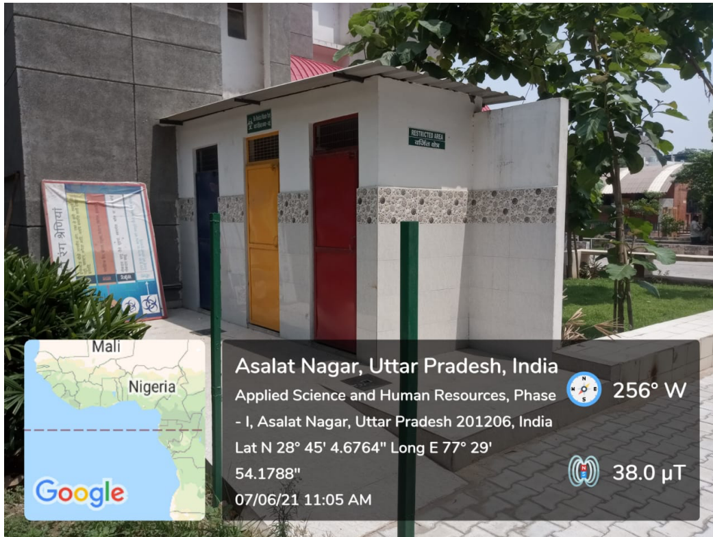
Biomedical waste segregation plant
